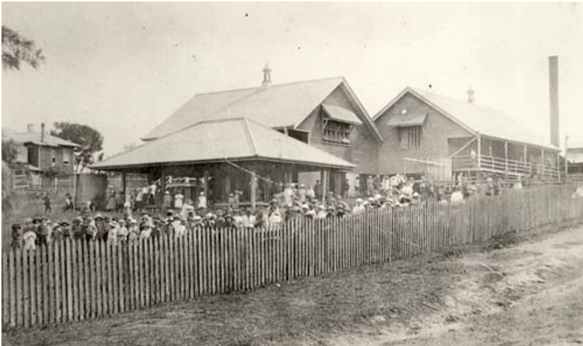
Figure 1. Nambour State School, Mitchell Street Nambour. ca. 1915. The School was located adjacent to the Moreton Sugar Mill. The mill chimney is visible on the far right and the head teacher's residence is pictured on the far left. Negative number: 87491. (Item held by John Oxley Library, State Library of Queensland, ca. 1915).
